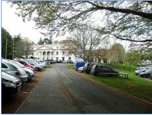
Follaton House, looking west
