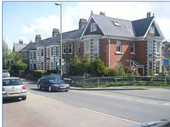
Early 20 th century terrace on the corner of lower Castle Street and Station Road, looking south-west
