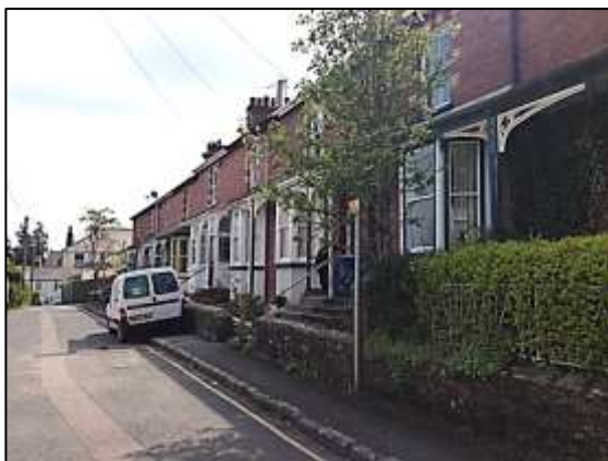
The south side of Belmont Terrace, looking east
