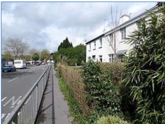
Late 20 th century terrace on Station Road bordering Borough Park, looking west
