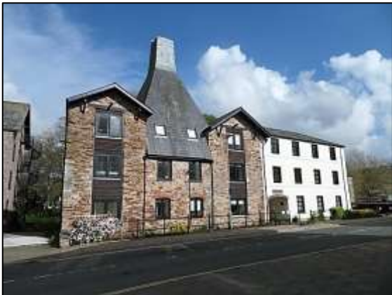
Former industrial buildings belonging to Symons Cider Factory on The Plains, now residential, looking east
