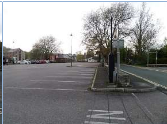
Car parking on Steamer Quay Road, looking north-west
