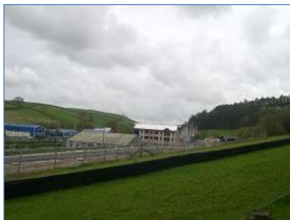
Baltic Wharf, looking south-east
