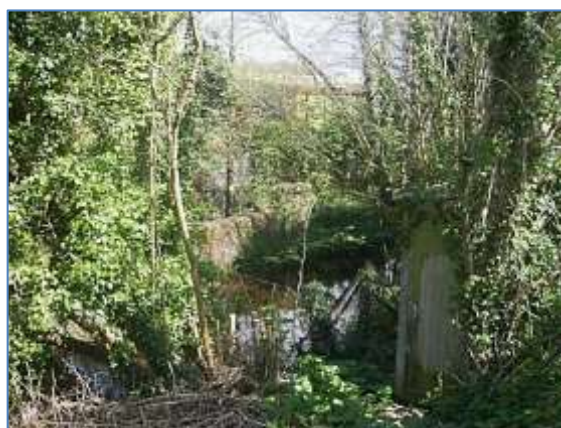
The culverted post-medieval mill leat at Broad Marsh, looking east from Totnes Station
