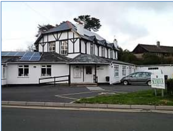
The former Cottage Hospital on Steamer Quay Road, looking east
