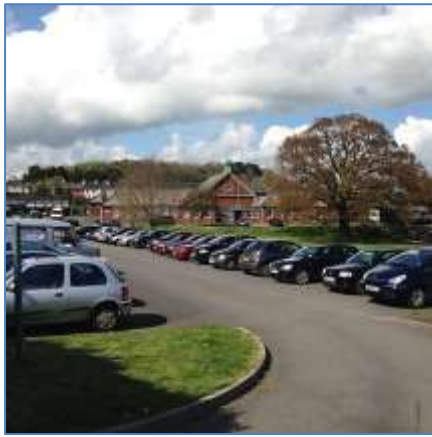
Former Totnes County School for Girls, now part of King Edward VI College, looking north-west
