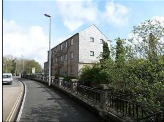
The 19 th century woollen mill and former granary, looking north-east
