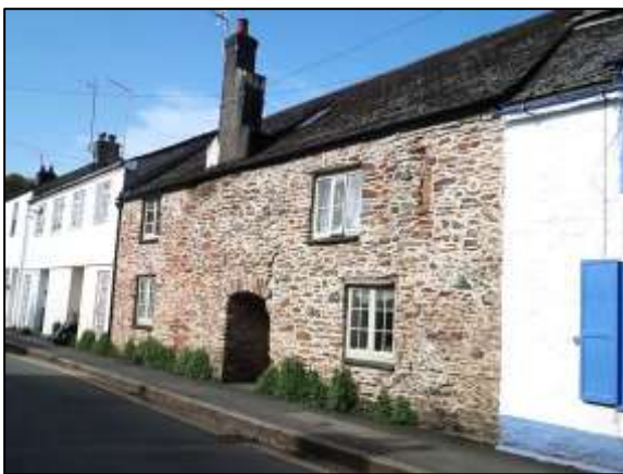
A 16 th century or earlier cottage at number 10 Warland, looking west
