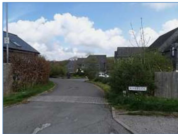
Riverside, looking north-east
