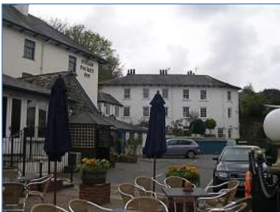
Steam Packet Inn, St Peter's Quay, looking west
