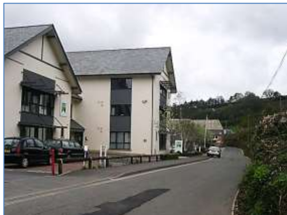
St Peter's Quay, looking south-east
