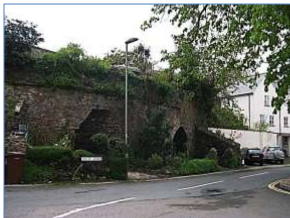
Section of wall and old limekilns on Shute Road, looking north-west from the present day St Peter's Quay
