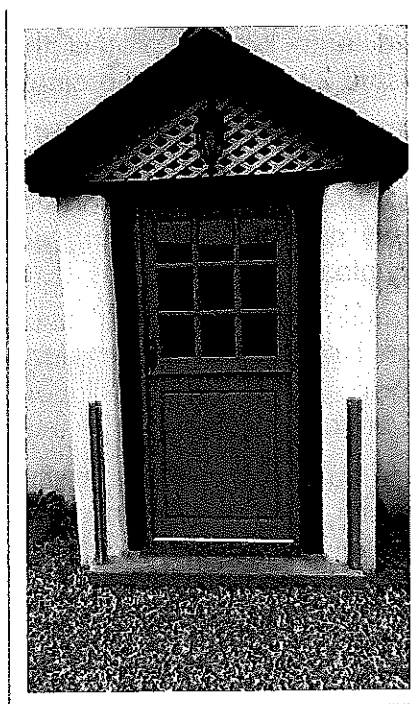
Property front door with slots either side, ready for flood boards to be slotted into place in the event of a flood warning – Umberleigh, North Devon
