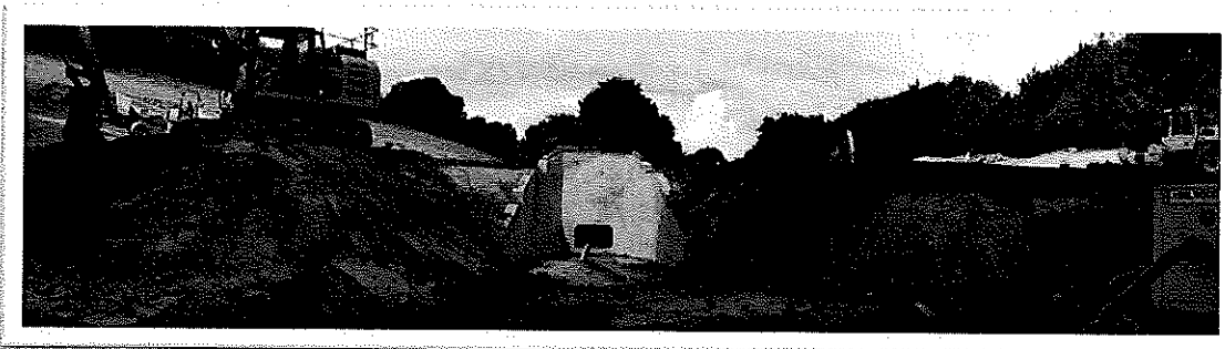
Looking south in Area 2, 2.5m tall with another 2.5m to be added to reach final crest level.
