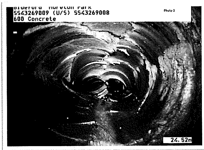
Condition of culvert prior to works commencing
