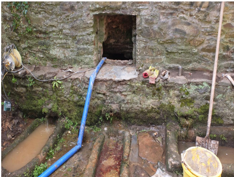
Fig.14 The channel beyond the dam is the last to be re-puddled.
