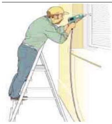
Incorrect – steps side on to work activity
