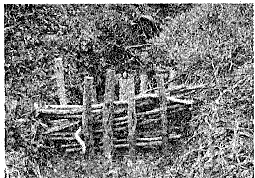
Any works within an ordinary watercourse channel will require Land Drainage Consent, such as this 'leaky dam.' Source: DCC Flood Risk Management Team
