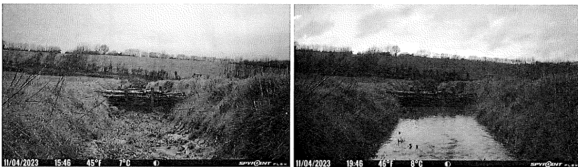
Leaky dams installed in the Chardstock areas as part of the Kit Brook Restoration Project. Source: Chardstock Eco-Group
