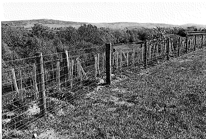
A Kested Hedge - a NFM intervention, to slow the flow of surface water. Source: DRIP
