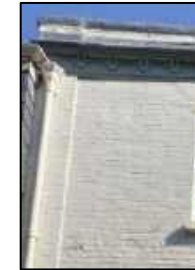
Brick with parapet
