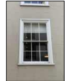
6 over 6 sash window
