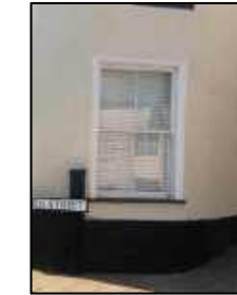
2 over 2 sash window
