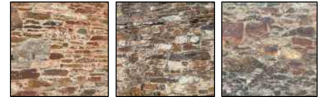
Local building stone.
