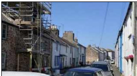
Building works undertaken Warland.
