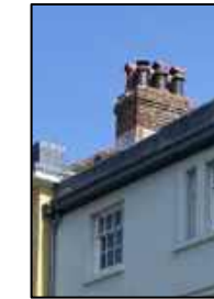
Endstack chimney
