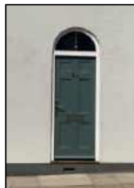
6 pane door with fanlight
