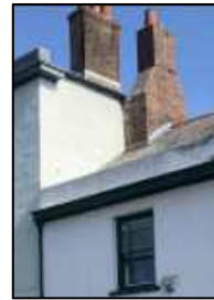
Endstack chimney
