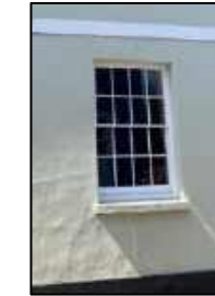
4 over 4 sash window
