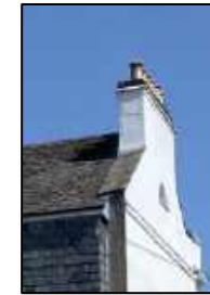
Endstack chimney
