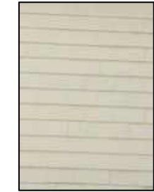
Painted hanging tiles
