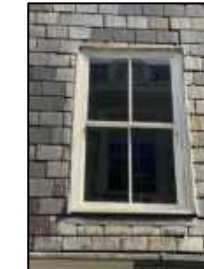
2 over 2 sash window
