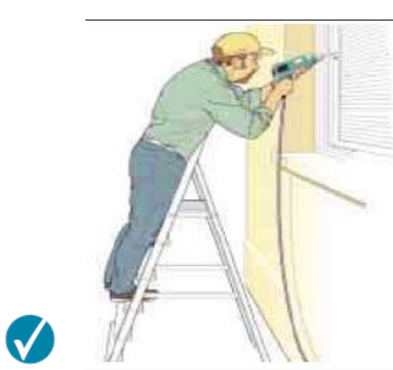
Correct – steps facing work activity
